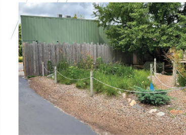
By using this area in the landscape, the space is now a rain garden that works with nature.
